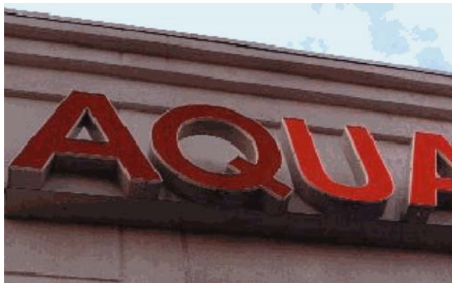
Fig. 1: The serviceman can usually locate the malfunctioning letters even in daylight. Notice how the "AQ" is darker than the "UA." In direct sunlight, inspect the neon by looking through the drain holes at the bottom of the letters.
